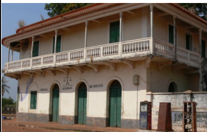
Bafatá Court before rehabilitation
